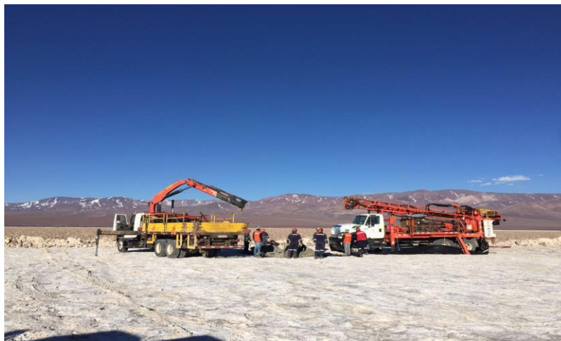
Figure 1: Drill Rigs on-site – Maricunga 28 September 2016
