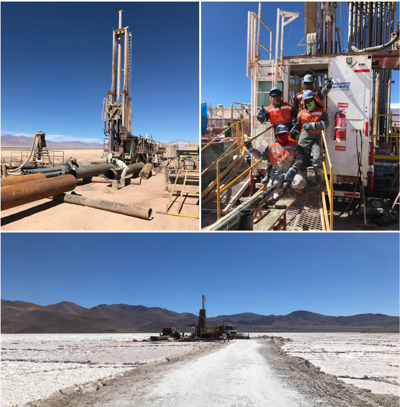
Figure 2.1, 2.2 & 2.3: Contractor Andinor’s construction of the 400m production well.
